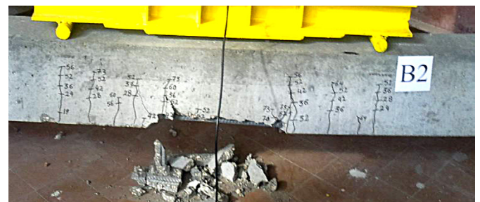
Fig. 5 Typical splitting failure for beam specimens without a confining transverse reinforcement.
